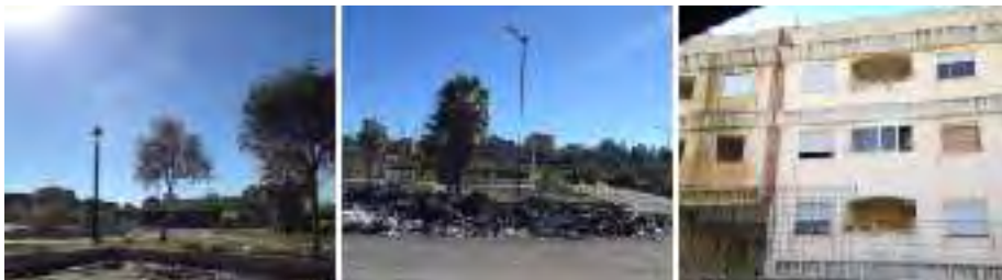
Fig. 6: Arghillà public spaces in decay (a), (b) and buildings (c) (Source: authors' photographs)
